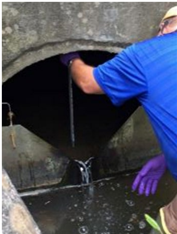
Figure 3.13. Storm water outfall monitoring
