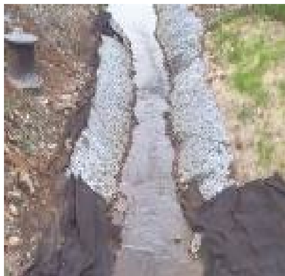
Figure 3.48. Construction of lined section of Mitchell Branch, MIK 0.7, in 1998
