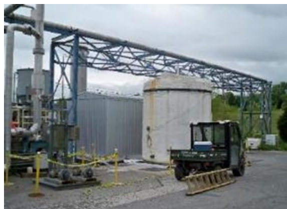
Figure 3.20. The Chromium Water Treatment System
