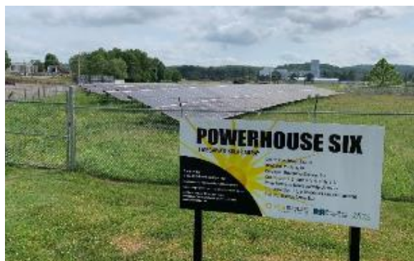
Figure 3.5. Oak Ridge Powerhouse Six Solar Farm
