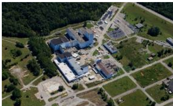
Figure 3.14. K-1200 Complex before decontamination and demolition
