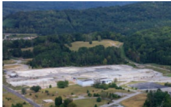
Figure 3.15. K-1200 Complex after decontamination and demolition
