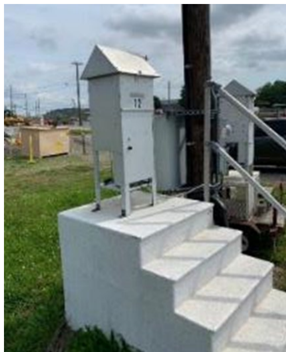
Figure 3.11. East Tennessee Technology Park ambient air monitoring station
